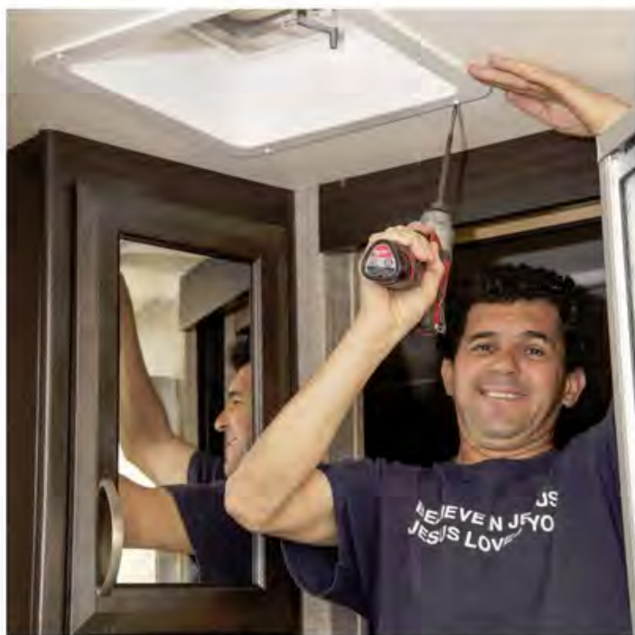
Service technician Romulo Demoraes installs an upgraded fan vent.
