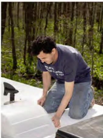
Demoraes removes a roof vent cap during an installation upgrade.
